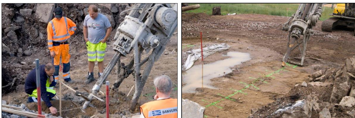
FIGURE 4.19 POSITIONING OF LIME CEMENT COLUMNS
