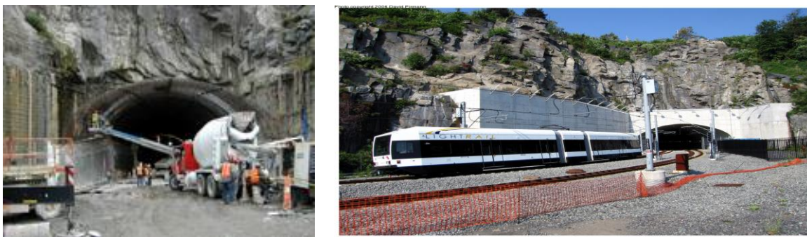
FIGURE 6.10. THE WEEHAWKEN TUNNEL IN NEW YORK WAS IN 2006 WIDENED FROM 8.4 x 6.4 M TO 19.7 x 10.4 M, SEE BERLINER ET AL (2004). PHOTOS BY JOHN PAPAS 2004 AND DAVID PIRMAN 2006.
