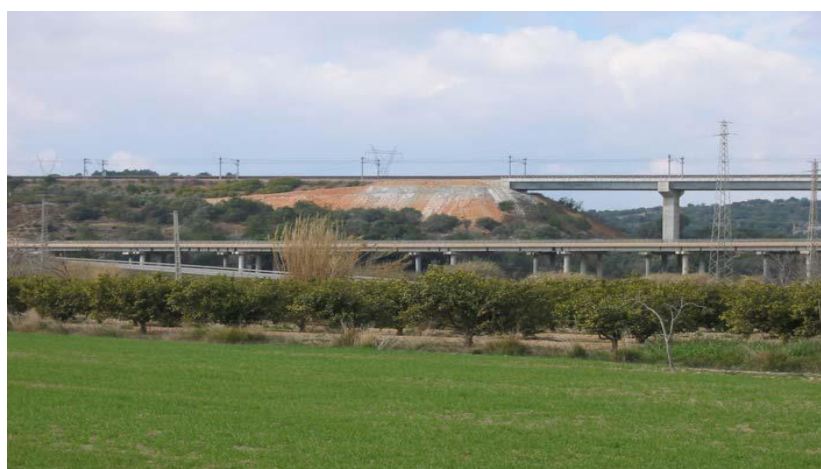
FIGURE 4.29. GENERAL VIEW OF THE EMBANKMENT WHERE THE SOIL IMPROVEMENT WAS ACHIEVED (EUROPEAN PROJECT SUPERTRACK, 2005)
