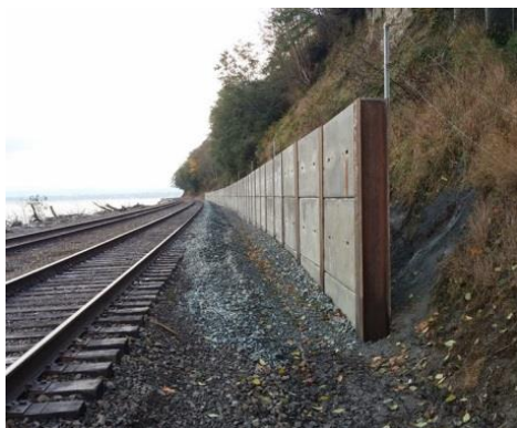
FIGURE 8.3. EXAMPLE OF RETAINING WALL TO PREVENT DEBRIS FROM LANDSLIDES, LABOE (2015).
