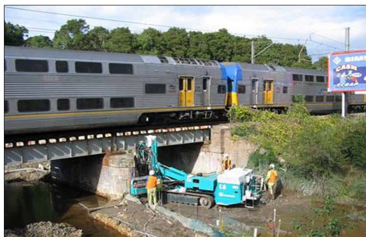
FIGURE 4.26. EXAMPLE OF VCC METHOD AT A RAILWAY BRIDGE
