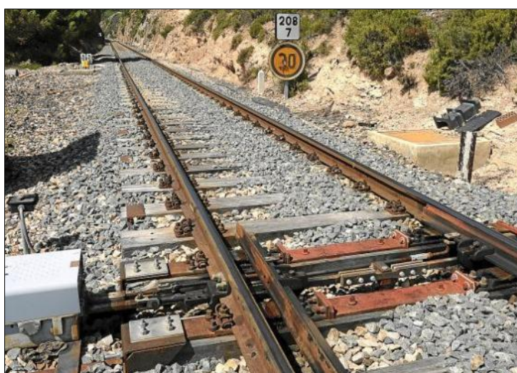
FIGURE 4.31 TREATED RAILWAY SECTION (ESCUDERO, 2011)
