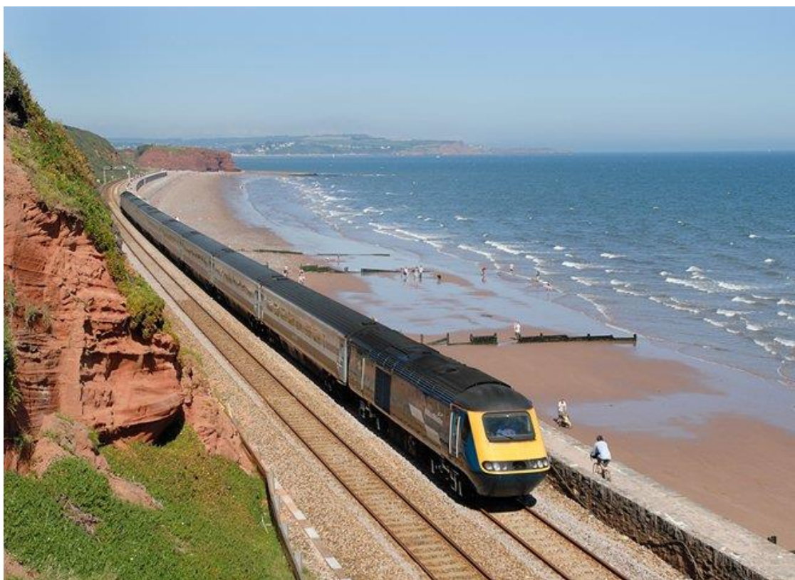
FIGURE 8.4. EXAMPLE OF A RETAINING WALL PROTECTING THE RAIL FROM THE SEA IN DEVON, U.K., SEE, SEA WALL RAILWAY (1845)
