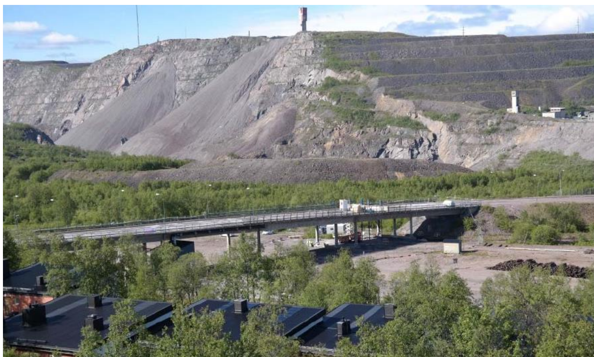
FIGURE 5.24 TEST TO FAILURE OF A STRENGTHENED PRESTRESSED FIVE SPAN BRIDGE IN KIRUNA IN 2014. OVERVIEW FROM N-E WITH THE LKAB IRON ORE MINE IN THE BACKGROUND. (BAGGE ET AL, 2014, 2015, 2016, 2017A,B)
