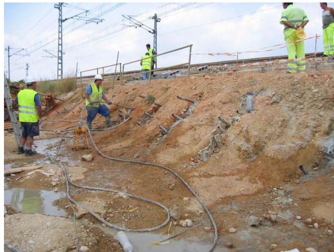
FIGURE 4.30. GROUTING OPERATIONS (EUROPEAN PROJECT SUPERTRACK, 2005)
