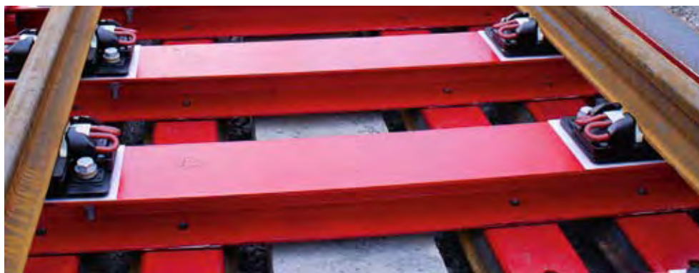
Figure 4.3.1-3: The steel frame in position prior to concreting
