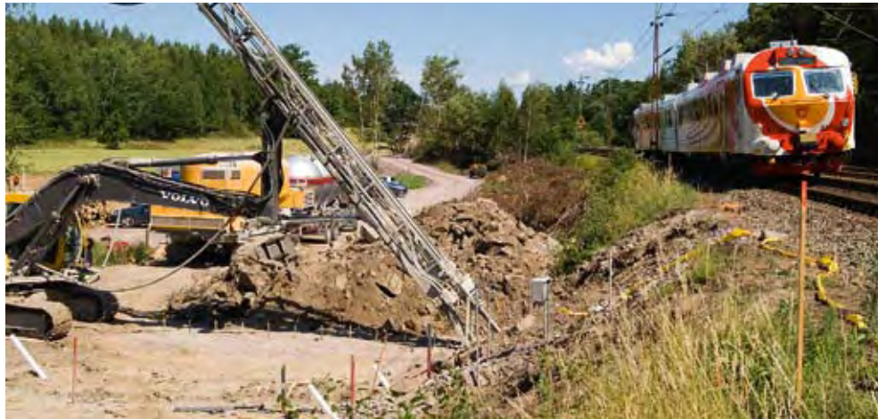
Figure 4.2.1-3: Installation of inclined lime cement columns under embankment
