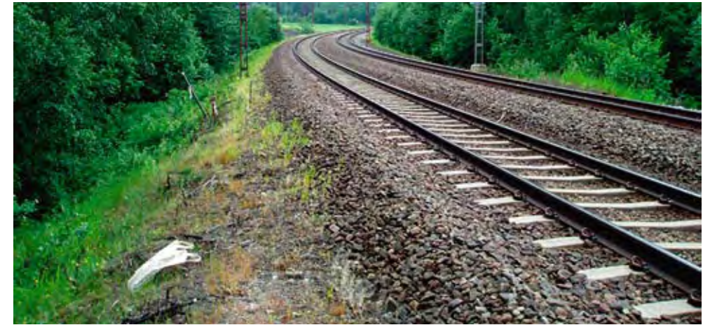
Figure 4.2.1-2: View of double track and embankment at Torp
