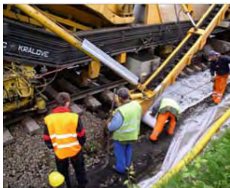
Figure 4.2.3-3: Old ballast removal with geocomposite installation
